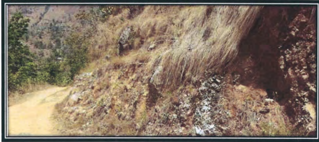
PHOTOGRAPH 2 EXPOSED ROCK SURFACES OBSERVED AT 6+600
